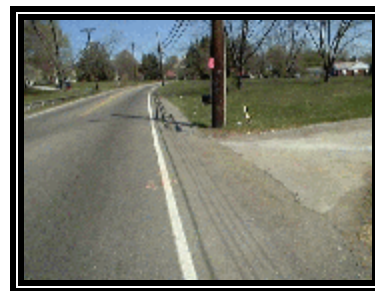
Figure 2: View of the utility pole.
