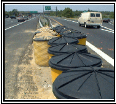
Figure 4. Placement of the sand barrel attenuators.
