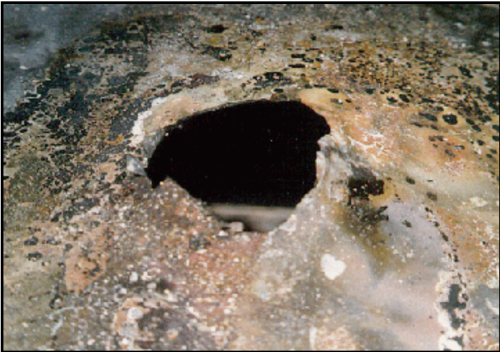
Figure 4. Close up of exit point.
