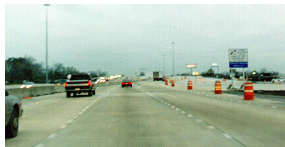
Figure 1: Case vehicle's southward travel path viewed from center lane of southbound roadway; Note: neither the farthest right (west) lane nor the road construction were present at the time of the crash (case photo #51)
