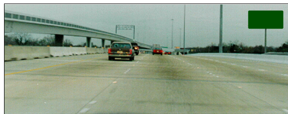
Figure 2: Approximate area of case vehicle's crash viewed from center lane of southbound roadway; Note: impacted concrete longitudinal barriers were located off both east (left) and west (right) sides of road and the farthest right (west) lane did not exist at the time of the crash (case photo #03)
