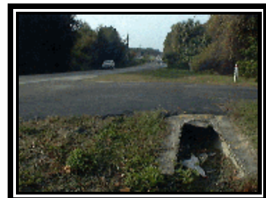
Figure 4. Struck driveway culvert.
