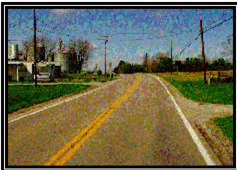
Figure 2: Westbound view 30 m (100 ft) from the POI.
