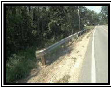
Figure 2. Guardrail impact area (end section replaced).
