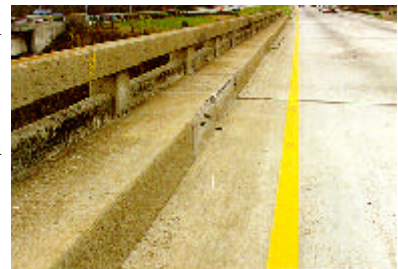
Figure 3. Ford Contour's impact with the barrier curb.
