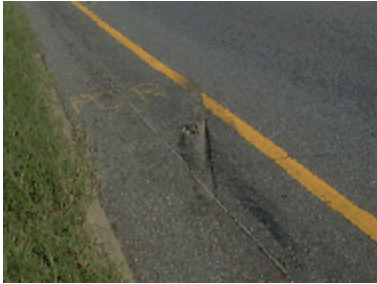
Figure 5. Left front wheel gouge in the asphalt shoulder.
