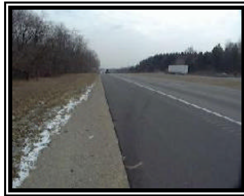
Figure 2. Look back view (east) from vehicle final rest showing post-impact yaw marks onto north shoulder.
