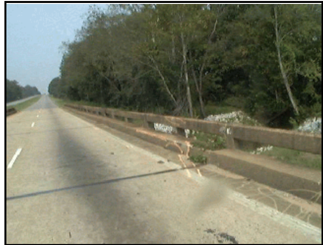
Figure 2. Point of impact with guard rail.
