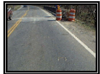
Figure 7. Struck bridge railing and final rest area of the Lexus.
