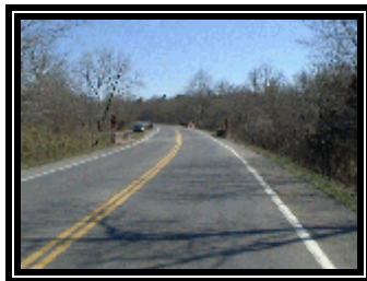
Figure 5. Area of initial departure from the eastbound travel lane.
