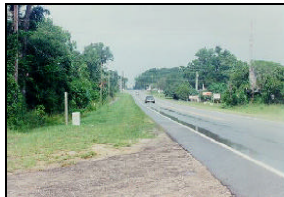
Figure 2: Case vehicle driver's view of eastbound traffic and intended left turn, looking west from mouth of driveway (case photo #02)
