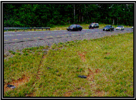
Figure 2: View of the marks through the median.
