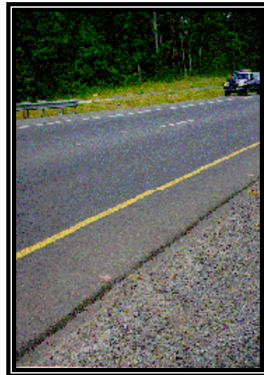
Figure 3: View of the rim impacts to the pavement edge.
