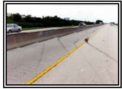
Figure 3. Tire marks to point of impact
