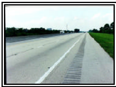
Figure 1. View looking north
