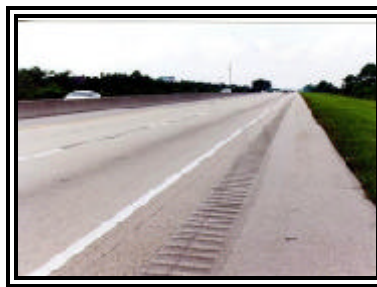
Figure 2. Tire marks on right shoulder
