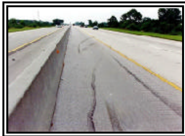
Figure 5. Post impact tire marks along median barrier
