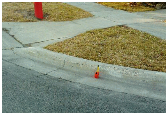
Figure 3: Case vehicle traveled off northwest corner of four-leg intersection striking first the curb (near tape measure) with its right front wheel and then the fire hydrant (case photo #04)
