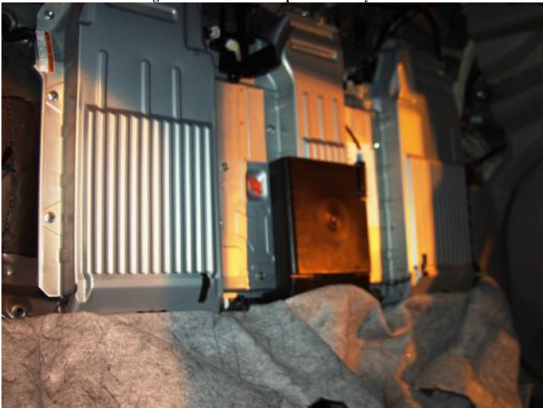
Figure A-36: Post-Test Propulsion Battery View
