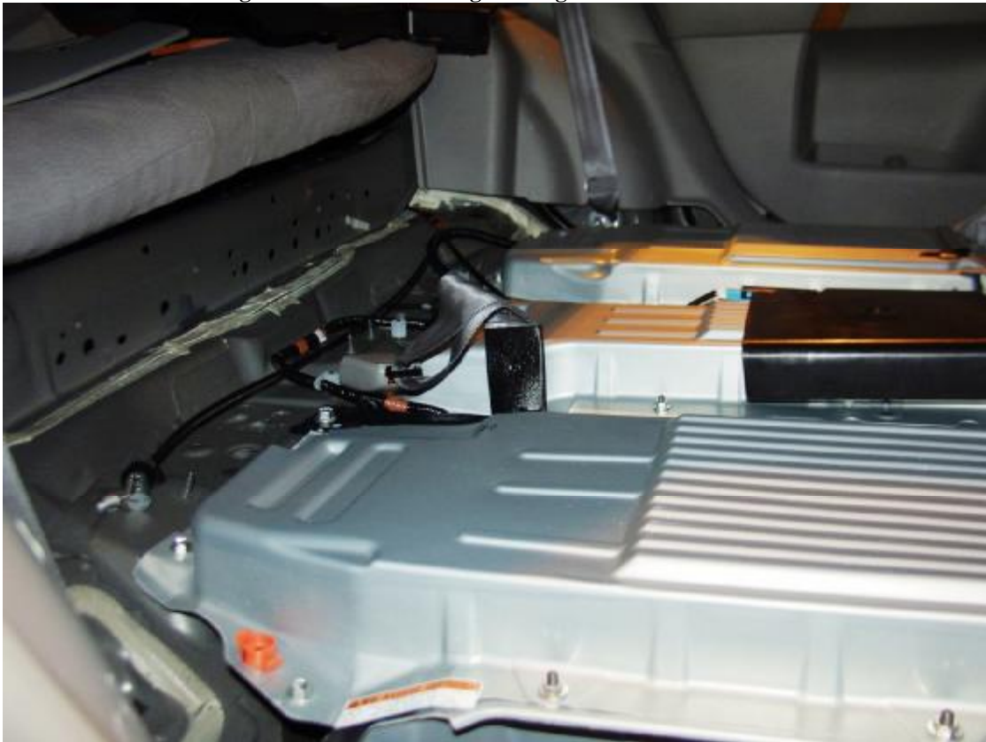
Figure A-38: Post-Test High Voltage Interconnect View
