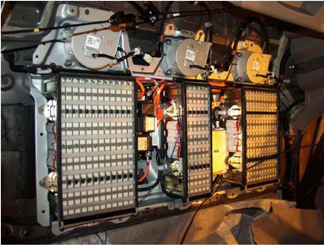
Figure A-35: Pre-Test Propulsion Battery View
