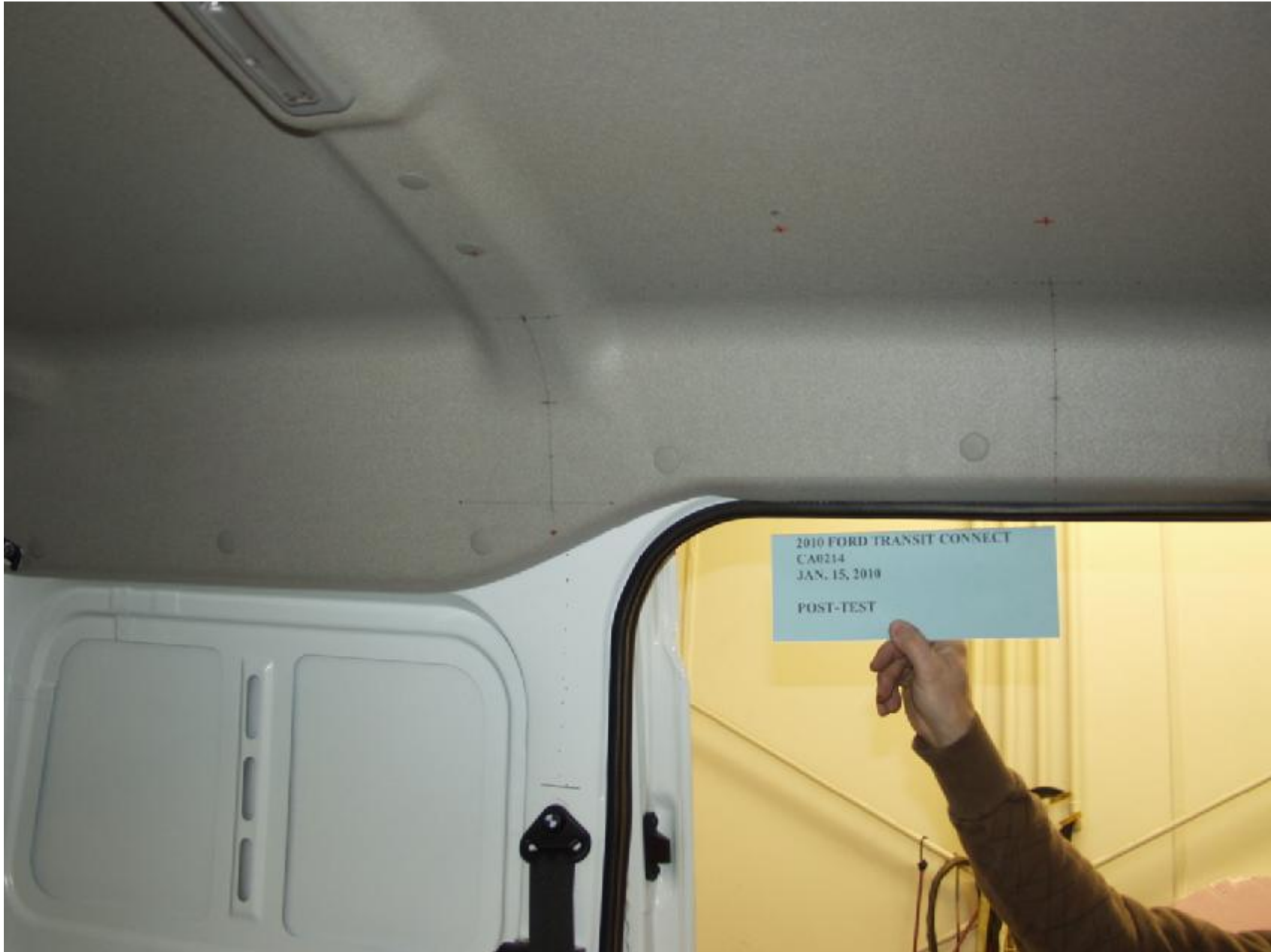
Figure A-24 : POST-TEST DRIVER SIDE OTHER PILLAR
