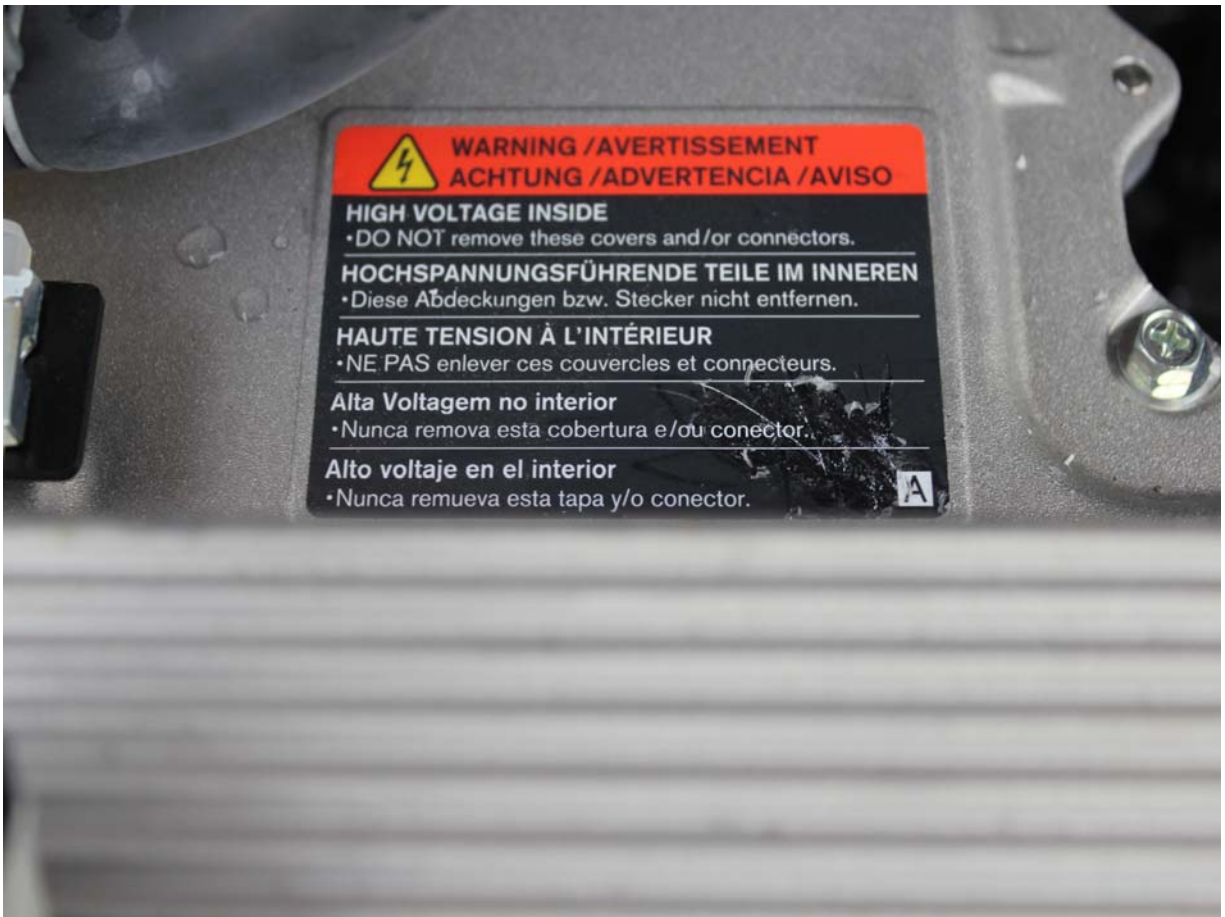
Drive Motor High Voltage Warning
