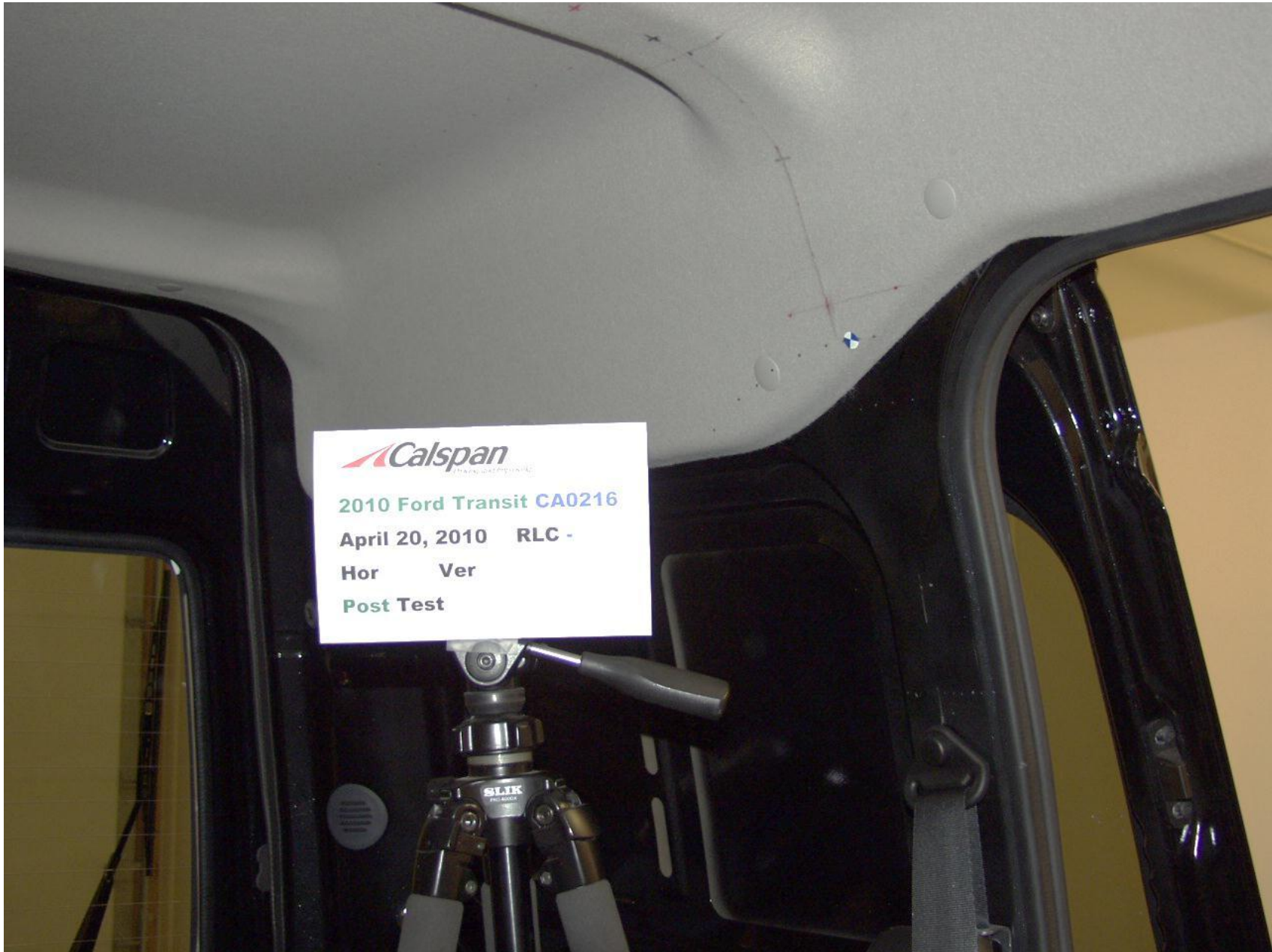
Figure A-22 : POST-TEST DRIVER SIDE OTHER PILLAR
