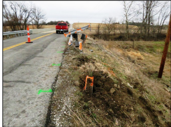
Figure 3: East-facing view of the damaged end treatment viewed from the area of initial impact.
