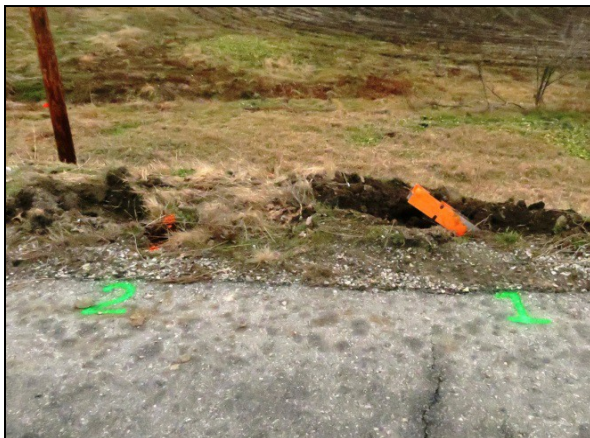
Figure 6: South-facing lateral view of the damaged end treatment and the locations of Post-1 and Post-2.
