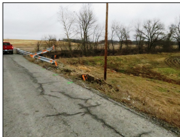
Figure 1: East-facing view of the crash site and damaged X-Lite guardrail system.
