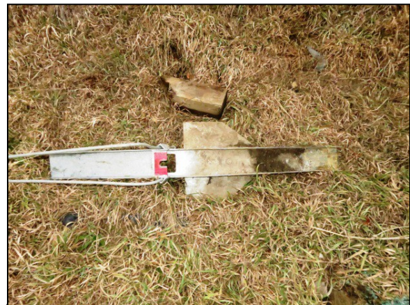
Figure 7: View of Post-2 at roadside, completely displaced from its original location.
