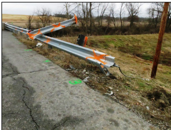
Figure 8: Overall view of the deformed X-Lite system at the time of the SCI inspection.
