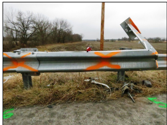
Figure 9: Lateral view of the displaced and deformed Panel-1 of the X-Lite guardrail end treatment system.
