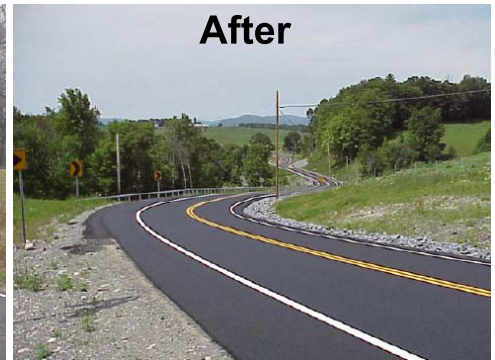
Roadside & visibility improvements; guardrail and delineation improved
