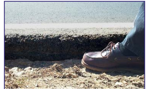
A vertical drop off such as the one shown in this photo is estimated at about 4-5 inches, which is considered a hazard if a driver’s vehicle slips off the pavement and onto an unpaved shoulder.
