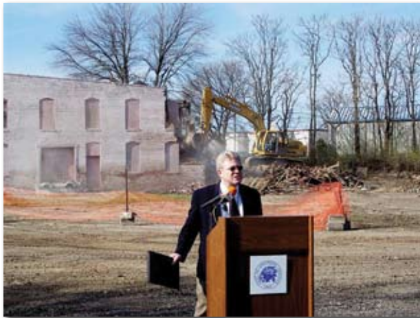
Demolition of the F.C. Cline Building
