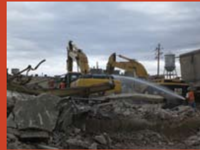
Demolition at Gates Rubber Plant, Denver, CO
