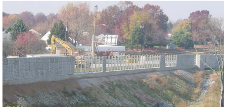
A barrier is the most common noise abatement measure. (Courtesy of FHWA)
