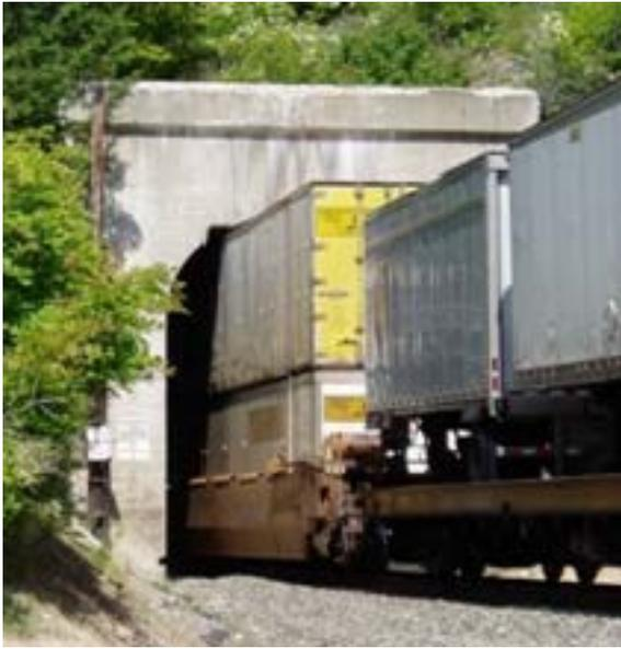
Notching tunnels allows double-stacked cars to pass through while retaining the historical integrity of the structure. (Courtesy of the National Gateway Clearance Initiative)
