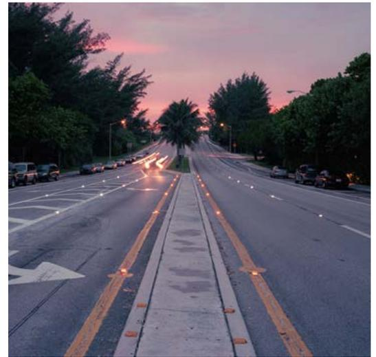
Embedded roadway lighting provides adequate illumination for vehicles and pedestrians and does not affect nesting areas. (Courtesy of FDOT)
