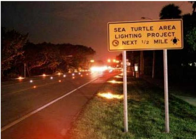
FDOT installed turtle-friendly, embedded lighting on State Road A1A (SR A1A) in a 2001 demonstration project. (Courtesy of FDOT)
