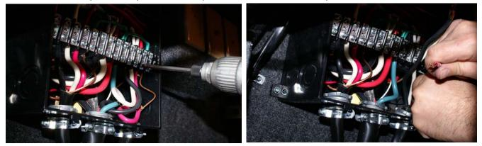
8. Remove the existing transfer switch from the compartment wall. Retain the mounting screws for re-use.
