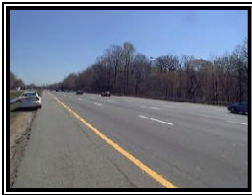
Figure 1. East view of travel lanes.
