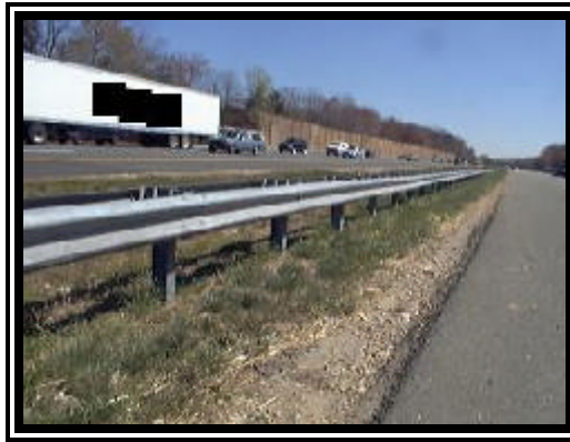
Figure 2. Impacted W-beam guardrail.
