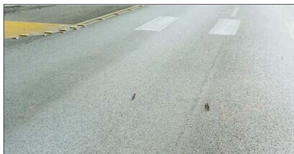
Figure 8: South-southeastward view of gouges in roadway's bituminous surface made by case vehicle's undercarriage as a result of its maximum engagement with Chevrolet pickup (case photo #04)
