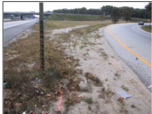
Figure 3. View of sign post from the sideswipe impact
