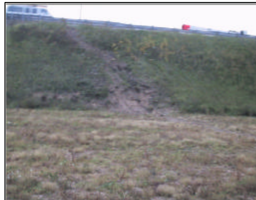
Figure 4. View of embankment
