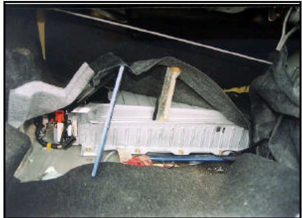
Figure 7. Battery pack in trunk—no spillage.
