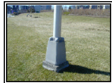
Figure 4. Replaced frangible base.
