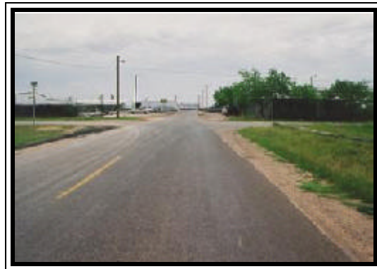
Figure 2. Eastbound approach for the 2000 Ford Taurus SE.
