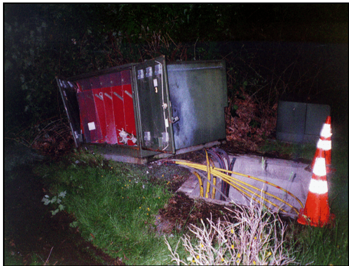
Figure 4. Damaged power transfer box
