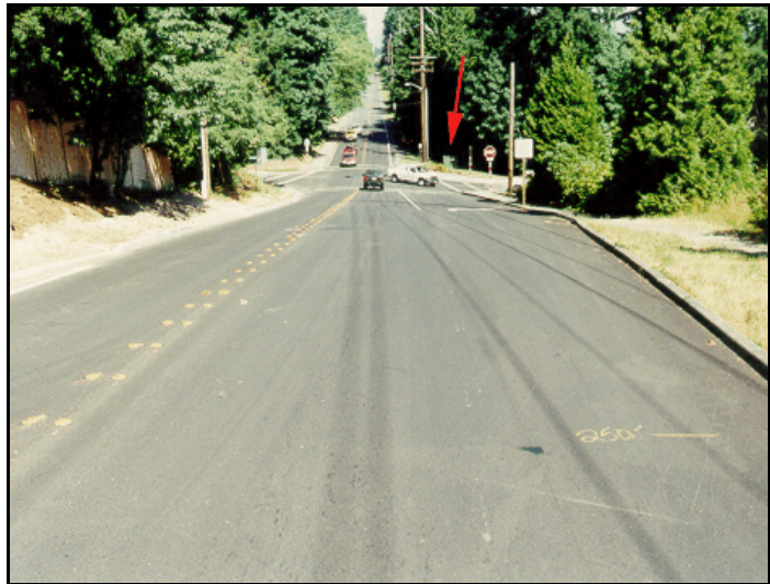
Figure 1. Downhill grade leading to impact areas
