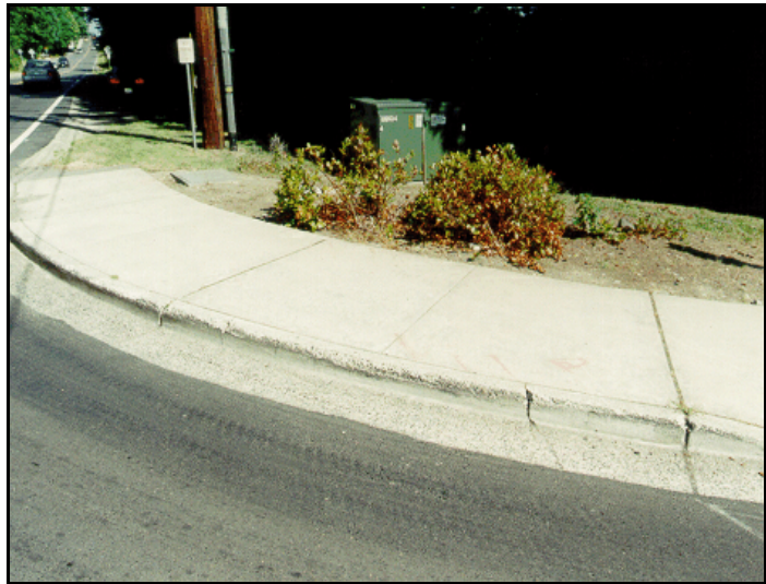
Figure 2. Impacts 1 and 2 with concrete curbs
