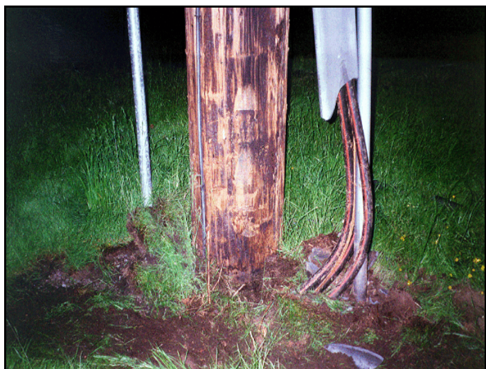
Figure 5. Damage to pole and electrical cabling
