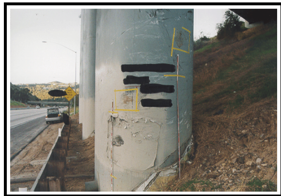
Figure 4. Struck concrete abutment. Occupant contacts are marked in boxes.
