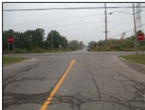
Figure 3. Westbound approach for the Saturn
