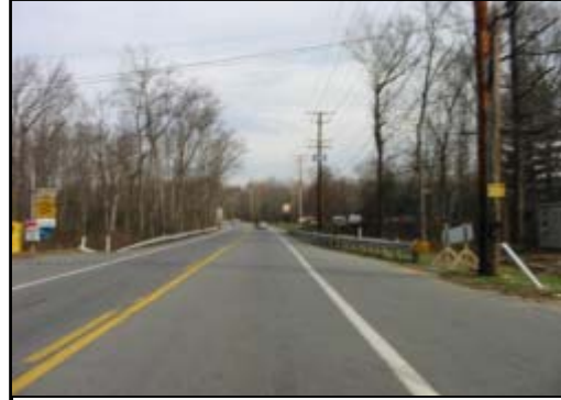
Figure 4. Area of impact from GMC's eastbound approach.
