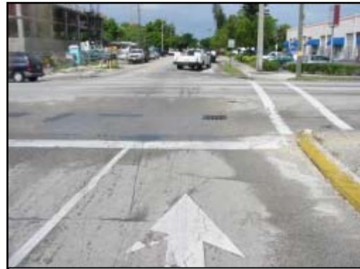
Figure 3. BMW approach to intersection.
