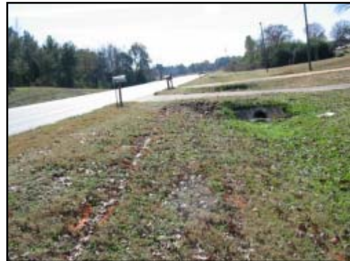
Figure 4. Area of impact between the Volkswagen and the first culvert.
