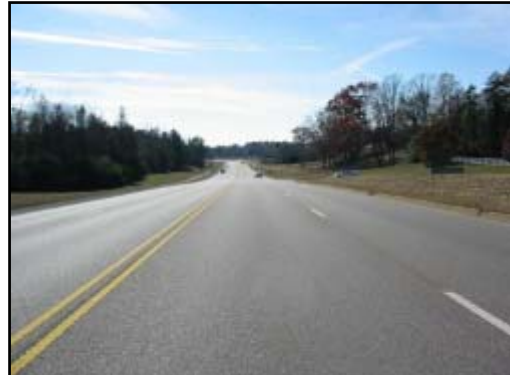
Figure 2. Southbound view of the crash site.
