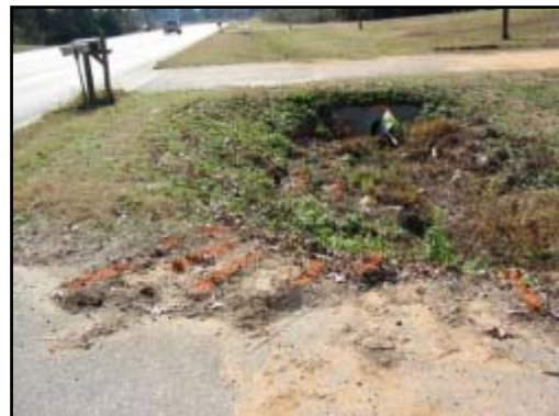
Figure 5. Second culvert impact and final rest for the Volkswagen.
