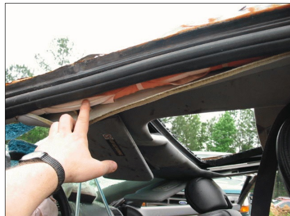
Figure 7: Case vehicle's exposed, non-deployed, left side-inflatable curtain air bag; Note: air bag exposed during rollover event as a result of damage to left "A"-pillar and roof side rail (case photo #37)
