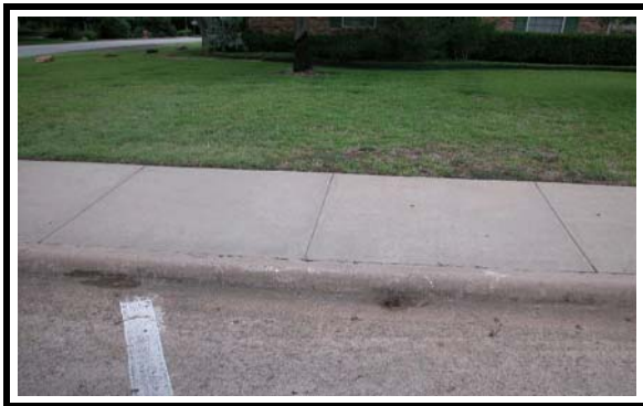
Figure 3. Close-up views showing curb impacts (Crash Events 1 and 2)
