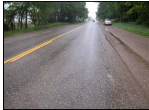
Figure 2. Southbound view of crash site
