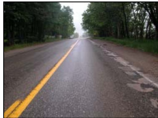
Figure 4. Northbound approach for the Ford Escort
