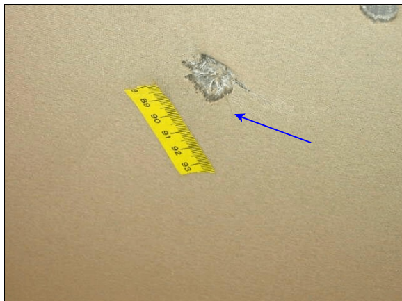
Figure 21: Close-up of contact (i.e., fabric gouge with hair) on roof surface over case vehicle's back seating area (case photo #54b)
