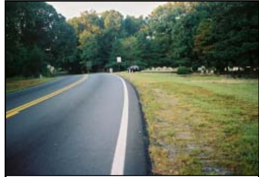
Figure 4. Southbound approach for the Grand Am
