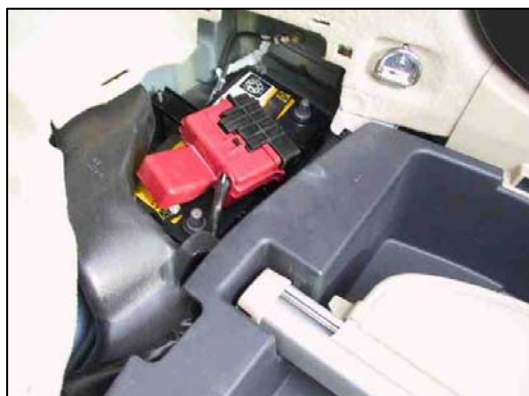
Figure 8 - Onboard battery system.
