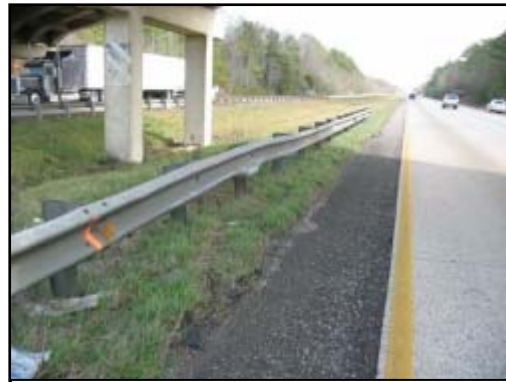
Figure 4. Impact to the second W-beam guardrail.
