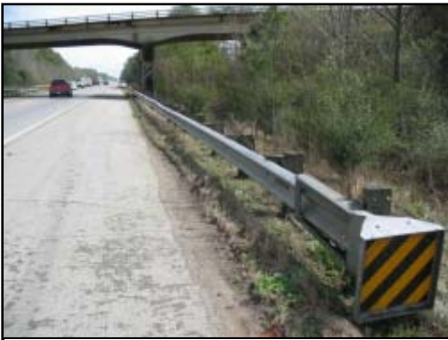
Figure 3. Impact to the first W-beam guardrail.
