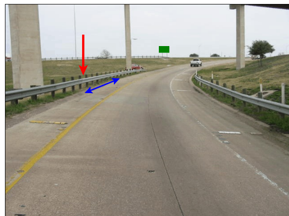
Figure 2: Case vehicle's northeastward travel path in rightward curving exit/entrance ramp; Note: oblique arrow indicates approximate point of impact and vertical arrow shows beginning of replacement guardrail (case photo #03)
