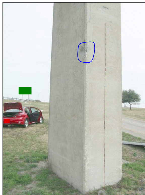
Figure 10: Case vehicle's contact area with bridge pillar; Note: height of contact area above ground and highlighted tire scuff mark (case photo #07)
