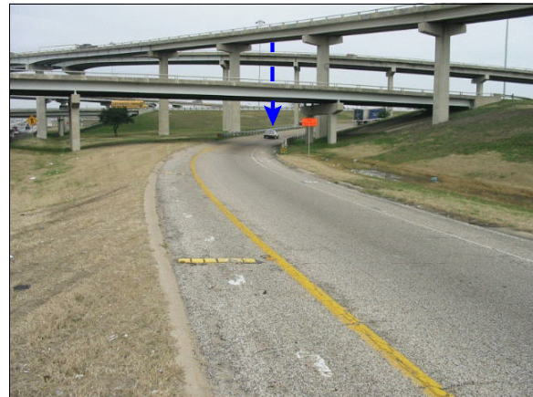
Figure 1: Case vehicle's north-northeastern travel path on exit/entrance ramp; Note: arrow indicates impact area (1 st event) with guardrail (case photo #01)
