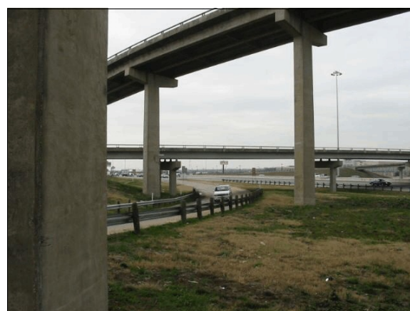
Figure 12: Southwesterly view from case vehicle's approximate final rest position of vehicle's north-easterly pre-crash travel path in right-hand curve in exit/entrance ramp; Note: distance from "W" beam guardrail to bridge pillar (case photo #10)
