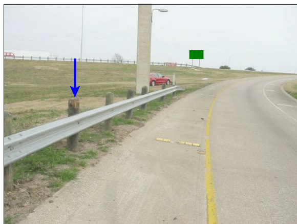
Figure 9: Case vehicle's area of roadway departure and contact with longitudinal barrier (i.e., "W" beam guardrail) located on northwest roadside of exit/entrance ramp; Note: unidentified tire mark on shoulder and arrow indicates suspected contact with guardrail support post (case photo #05)
