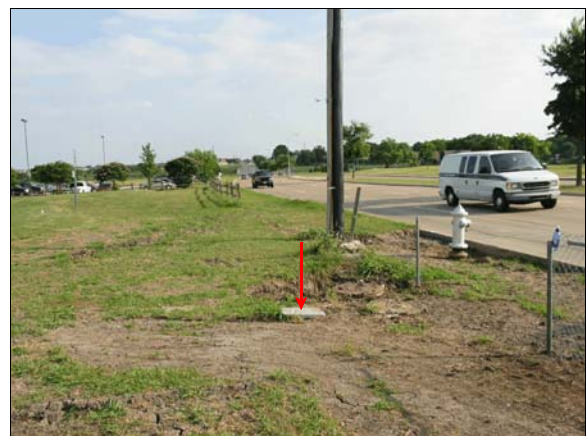
Figure 6: View to southwest showing damage to woven wire fence, missing section of wooden fence, water main cover (arrow), fire hydrant and area of rest of case vehicle (near bottom of photo)
