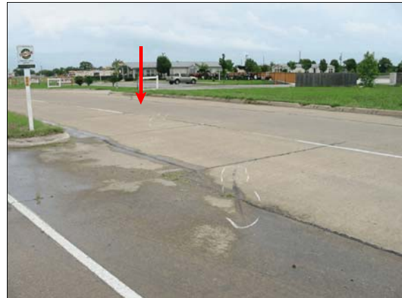
Figure 3: Overview of area of rollover across service roadway, plastic and/or rubber transfer from case vehicle's luggage rack and/or right door gasket highlighted in white in foreground, arrow shows area of final rest
