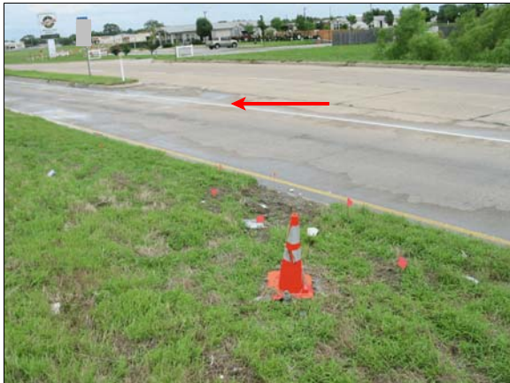
Figure 2: Orange cone shows base of luminaire pole impacted by case vehicle, photo view to southeast, arrow shows area of rollover
