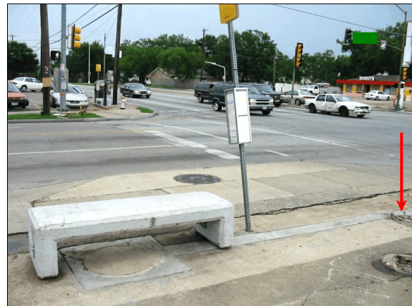
Figure 14: East-southeast view from case vehicle's approximate final rest position; Note: arrow indicates approximate impact with post and this contractor believes southeast corner of bench was on south side of bus stop sign post at time of crash (case photo #08)
