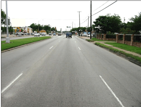
Figure 1: Case vehicle's westbound travel path in center through lane of western roadway of divided city trafficway (case photo #01)
