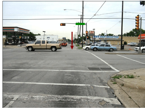
Figure 5: Chrysler's northern travel path in outside northbound lane just prior to four-leg intersection; Note: arrow shows approximate area of impact (case photo #13)
